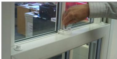
To open the bottom sash, raise the sash using the lift handles.
