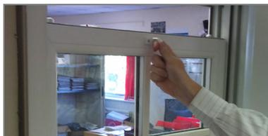
To close and lock, close both sashes by reversing the procedures above, then close the lock by turning the lever clockwise. Finally, lock the window with the key supplied.
