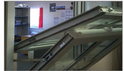
After cleaning, close the top sash by using both hands to push it firmly but carefully back into its upright position. Make sure that the latch knobs click back in to position to hold the top sash in place.
