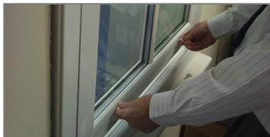
To open the top sash, lower the sash using the ring pull handle.
